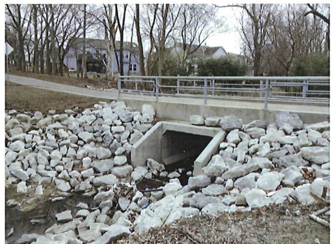
Completed Low Water Crossing - Eudora Walking Trail
