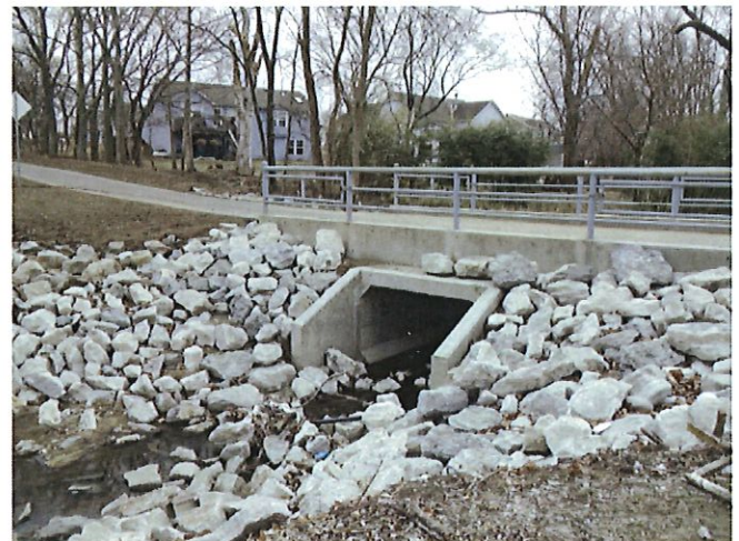
Completed Low Water Crossing - Eudora Walking Trail
