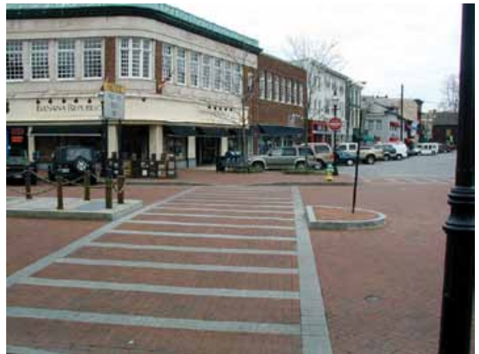
The “zebra” crosswalk is an adaptation of the ladder design, created to keep pedestrians together where they can be seen by motorists and cross the street more safely. (Photo courtesy of Dan Burden)
