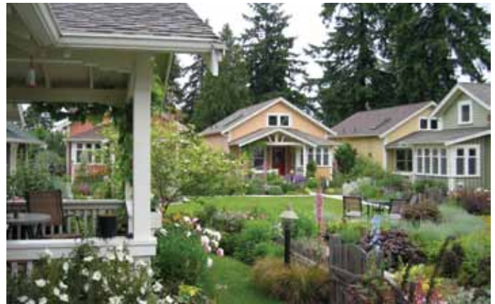
Third Street Cottages consist of eight detached, one-bedroom-plus loft cottages clustered around a garden courtyard with detached parking. The city of Langley, Wash. (pop. 1100), was the first to adopt an innovative “Cottage Housing Development.” (Photo courtesy of Ross Chapins Architects)
