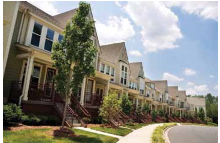
Sycamore Green, located in Charlotte, N.C., is a residential development designed to integrate low-income residents into a market-rate apartment complex. (Photo courtesy of Stewart Engineering)
